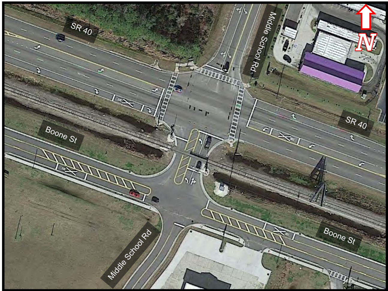
Figure 67. Middle School Road at SR 40 Intersection
