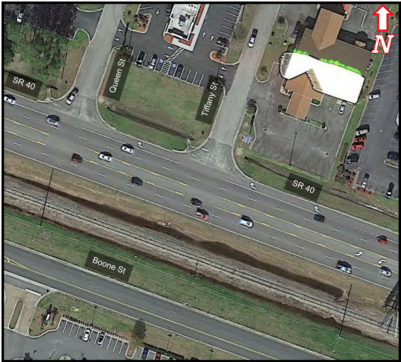
Figure 59. Tiffany Street at SR 40 Intersection
