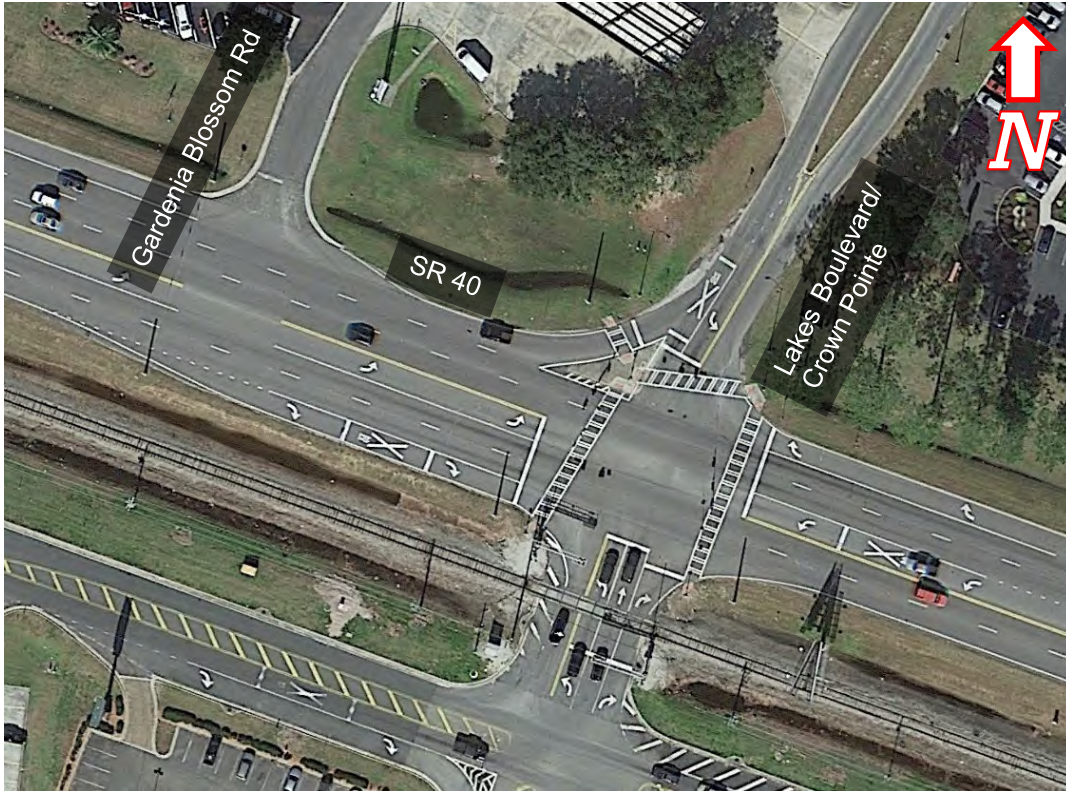
Figure 14. SR 40 from Gardenia Blossom Road to Lakes Boulevard/Crown Pointe Parkway
