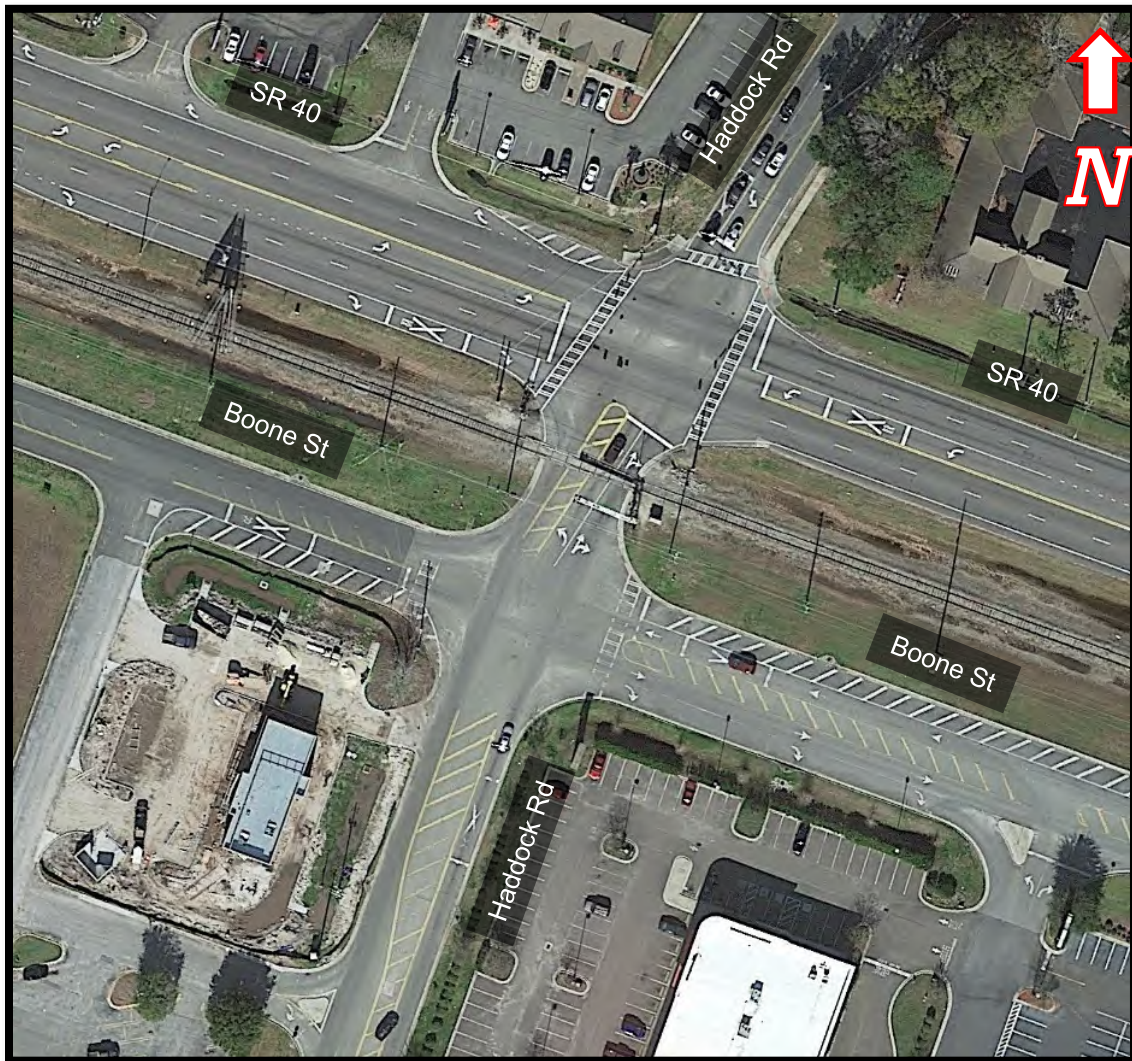
Figure 77. Boone Street at Haddock Road Intersection
